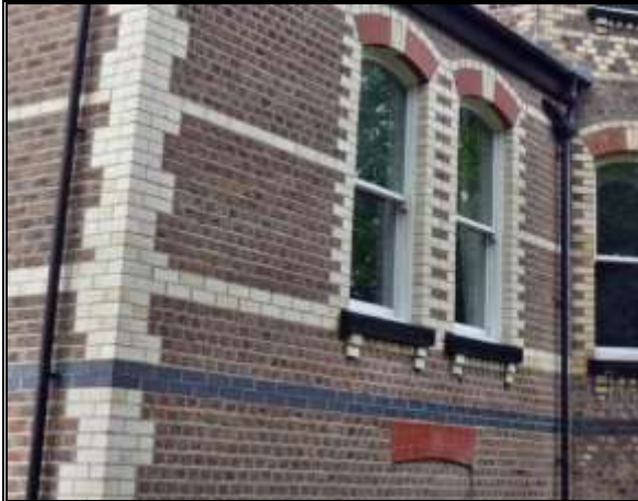
Photograph 10: Polychromatic Brickwork and Header Bond
