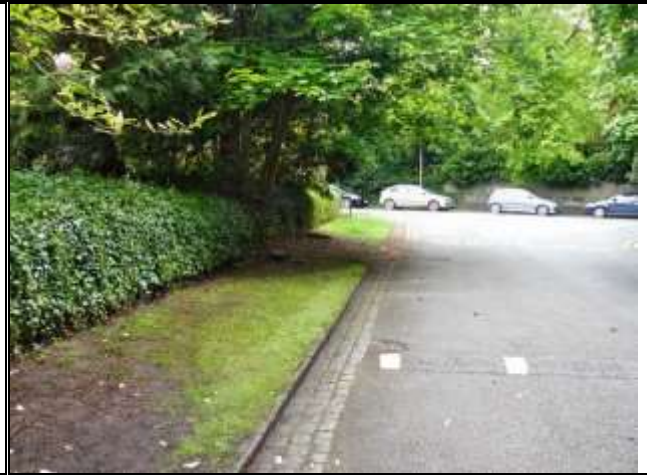
Photograph 124: Boundary Wall with Overgrown Ivy, Parkfield Road
