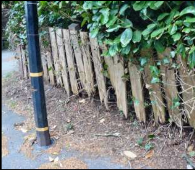
Photograph 119: Timber Fence along Charcoal Road
