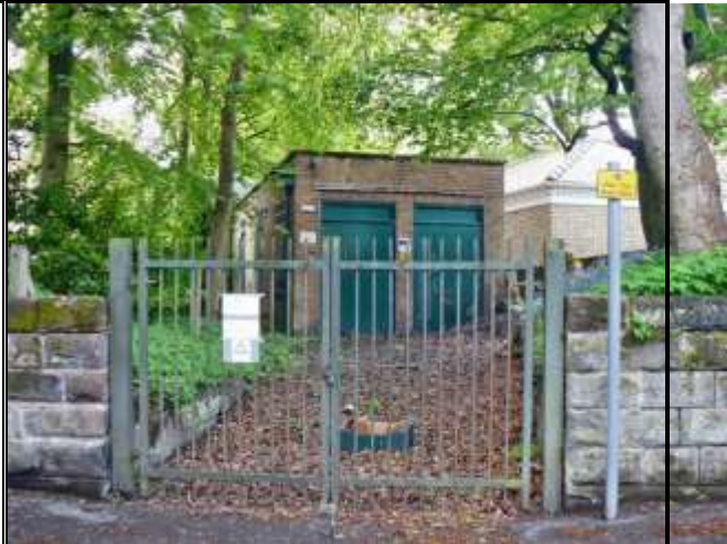
Photograph 27: Electricity Substation, Booth Road
