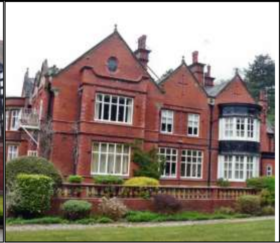
Photograph 87: Victorian Property with Decorative String Courses and Hood Moulds, Charcoal Road
