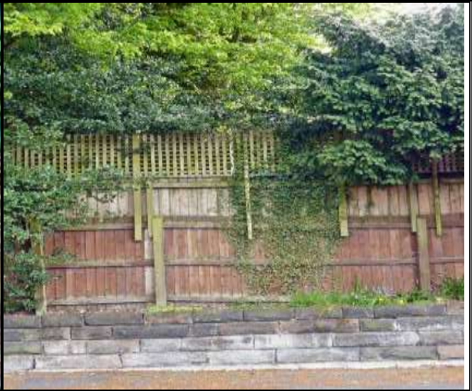
Photograph 120: Inappropriate Boundary Treatment along Oldfield Road
