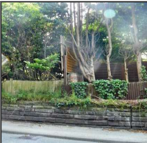
Photograph 114: Combination of Boundary Treatments along Dunham Road.
