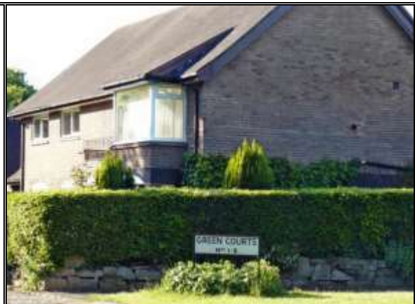
Photograph 71: Functional Style with Minimal Architectural Detailing, Green Courts
