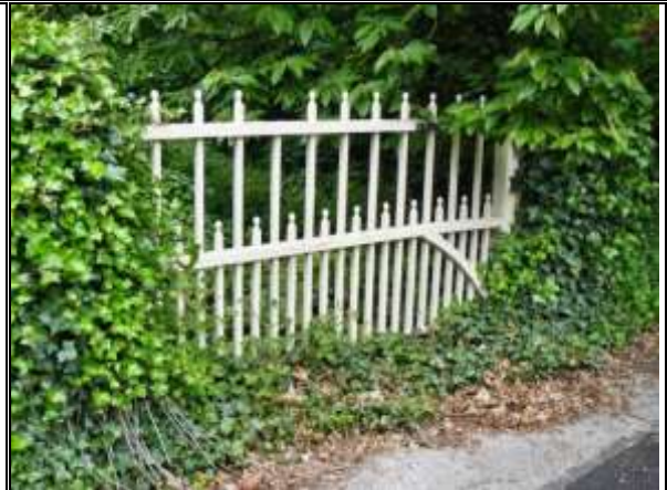
Photograph 49: Gate and Gateposts (under Ivy) of Former Carriageway
