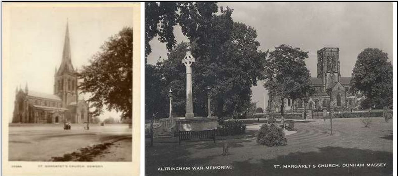
Photographs 1 & 2: St. Margaret's as built (Altrincham Area Image Archive, BM0250) and after 1927 with War Memorial (Trafford Lifetimes, TL8815)
