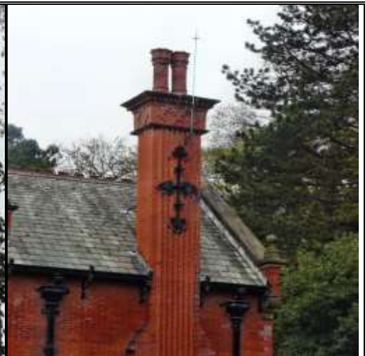
Photograph 89: Roof with Ridge Tiles, Finials and Chimney Stack
