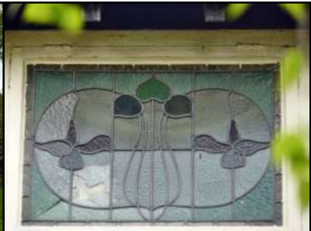
Photograph 13: Stained Glass Windows to Birchdale on Bonville Road
