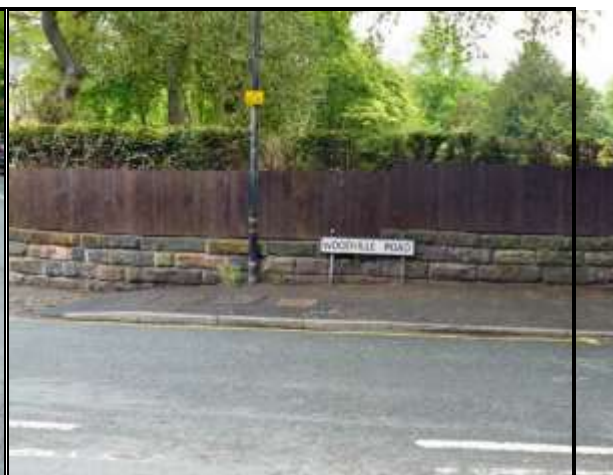
Photograph 29: Stone Wall with Fencing Above, Groby Road
