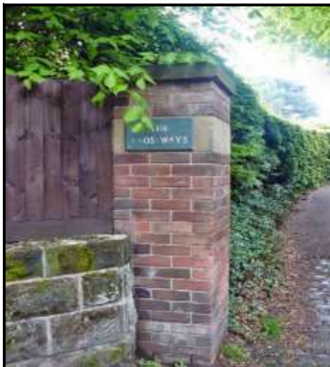
Photograph 121: Modern Replacement Gate Post, St Margaret's Road
