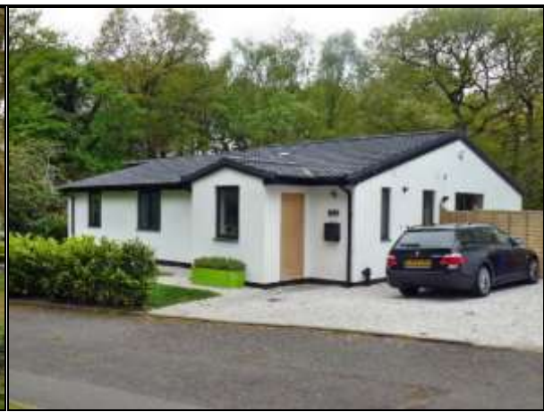
Photograph 95: Modern Bungalow, Next to the Reservoir
