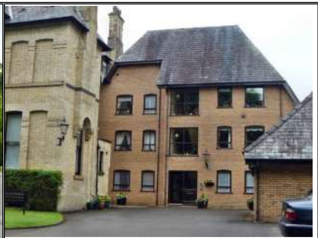
Photograph 132: Extension to Inglewood, St Margaret's Road
