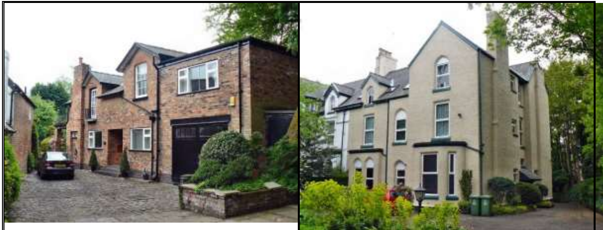
Photograph 14: UPVC Replacement Windows to Grove Cottage
