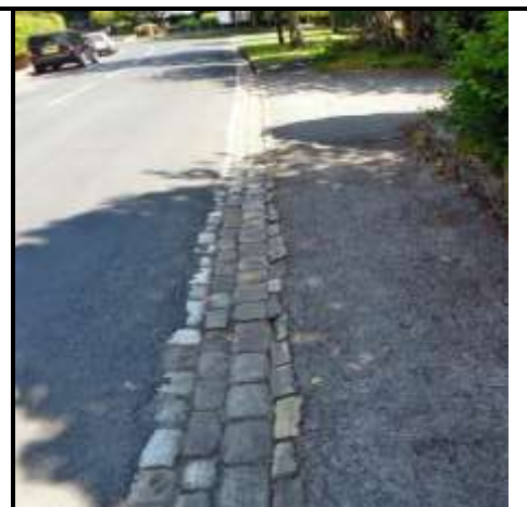
Photograph 79: Setts, Bow Green Road
