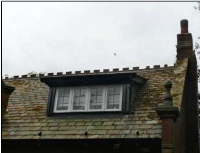
Photograph 88: Ridge Tiles and Finials
